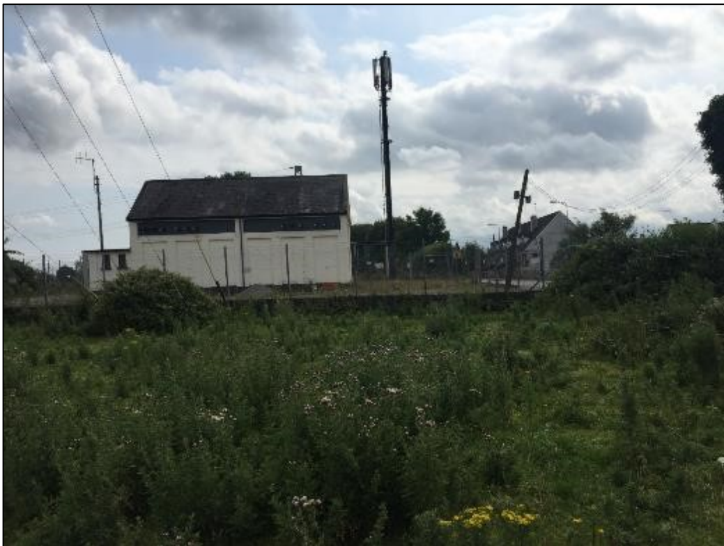
Plate 6: View of Ashe Road substation from west
